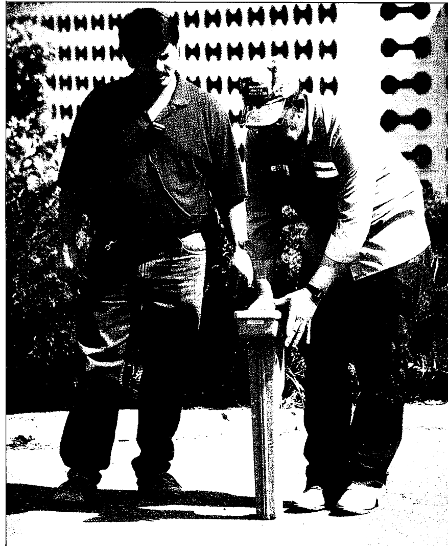
The locating operator is able to track the direction of the bore using the subsite locator.
