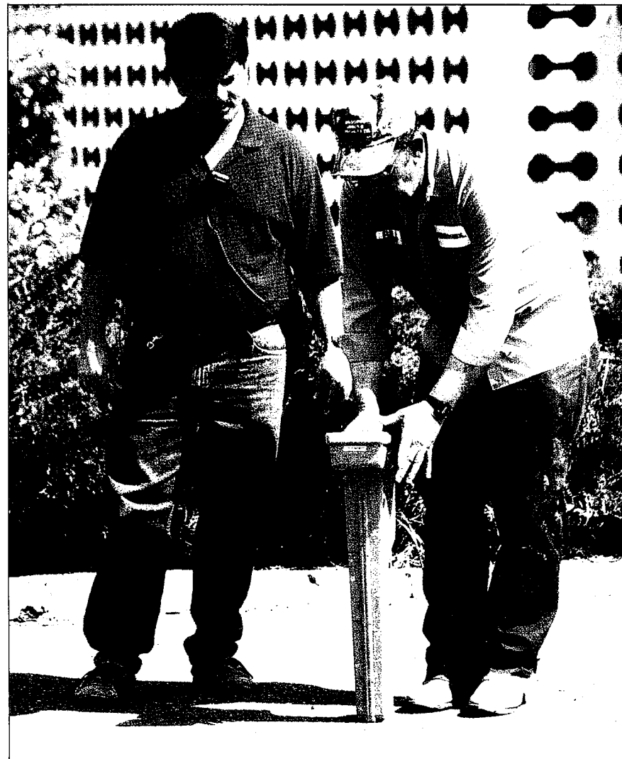
The locating operator is able to track the direction of the bore using the subsite locator.
