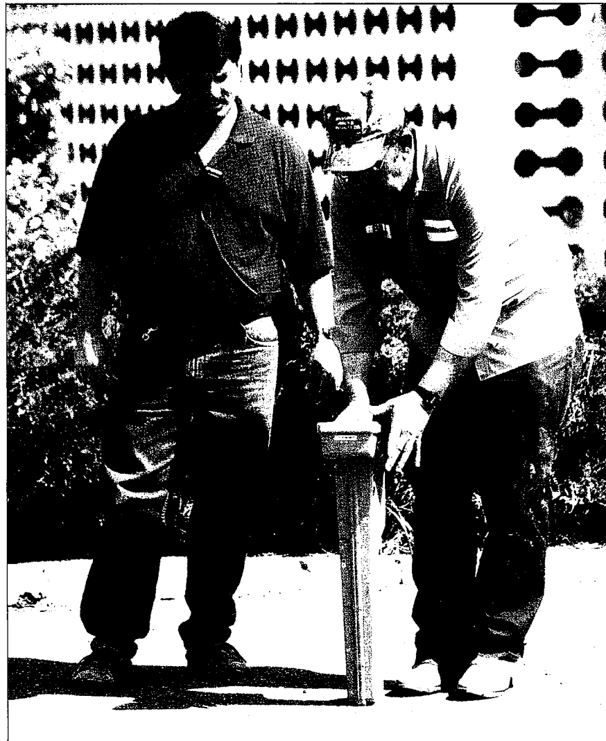
The locating operator is able to track the direction of the bore using the subsite locator.
