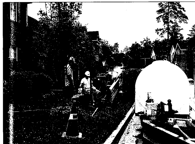
Damage to yards and landscaping was minimized using self-contained directional boring systems, which allowed the contractor to work in tight areas.
