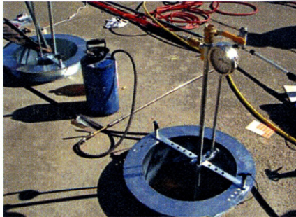
Left: STM(s) being completed with keyhole tools and apparatus. Right: Completed STM connection.
